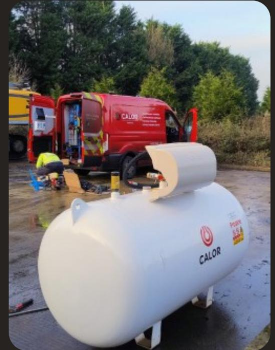
Transition to cleaner fuel for our remaining gas forklift fleet through the installation of a bulk tank
